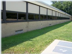
Shaler Area Elementary School- Original Windows.
