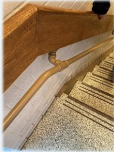
Burchfield Primary School- Stair Guard rails.
