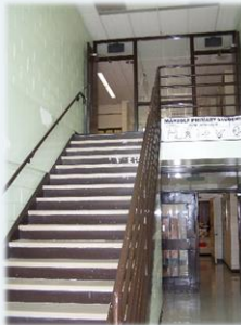
Marzolf Primary School- Stair Guard rails.
