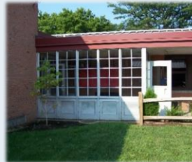
Burchfield Primary School- Aluminum Entrances.
