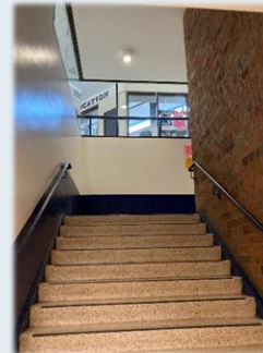
Shaler Area High School -Stair Treads.
