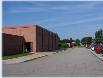
Marzolf Primary School-Entrance.
