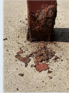
Burchfield Primary School -Canopy Columns.
