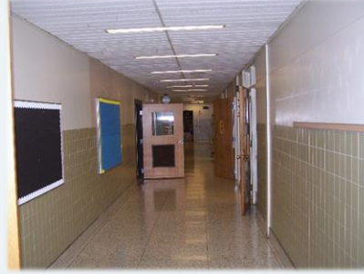
Marzolf Primary School-Dead end corridors.
