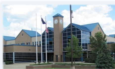
Shaler Area Middle School- Entrance Security Vestibule.
