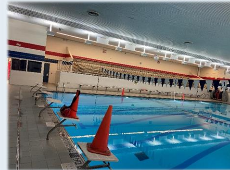
Shaler Area Elementary School – Inaccessible Spectator seating.
