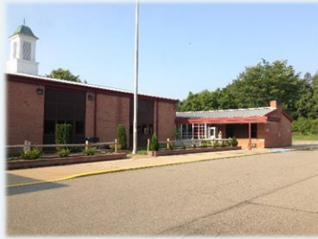
Burchfield Primary School- Entrance.
