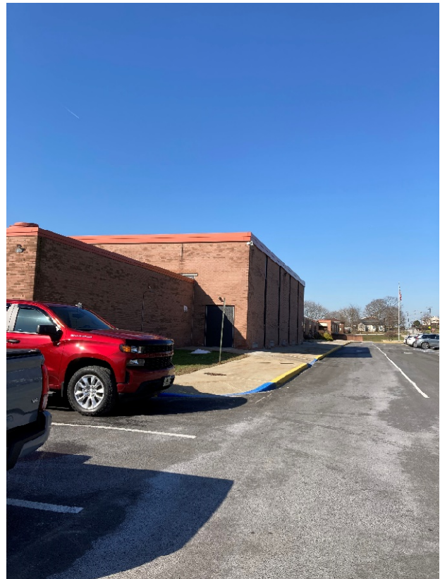
Marzolf Primary –Exit from Gymnasium.
