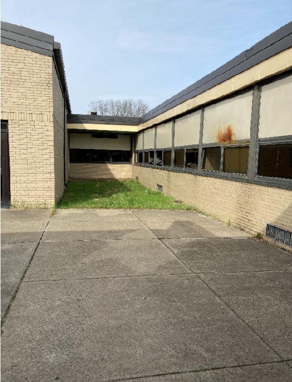
Building's exterior windows leak air and water at their perimeter and are in poor condition.
