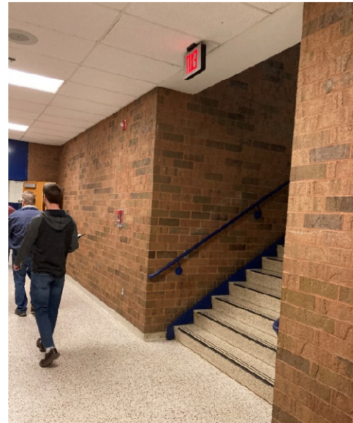
New rubber tread and risers need to be installed throughout the building.
