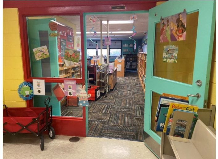
Shelving and tables in library need to be replaced.
