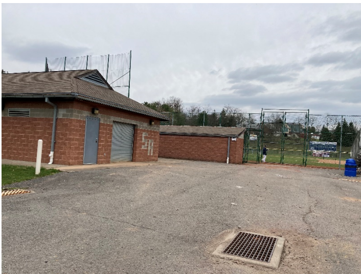
Athletic field support buildings roofing /fascia soffits, downspouts need to be replaced.
