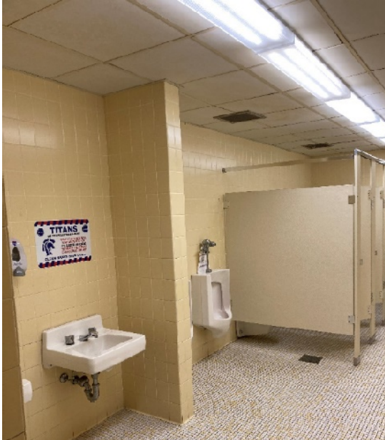
Non-compliant lavatories, sinks and toilets do not provide adequate accessibility clearances at the fixtures.
