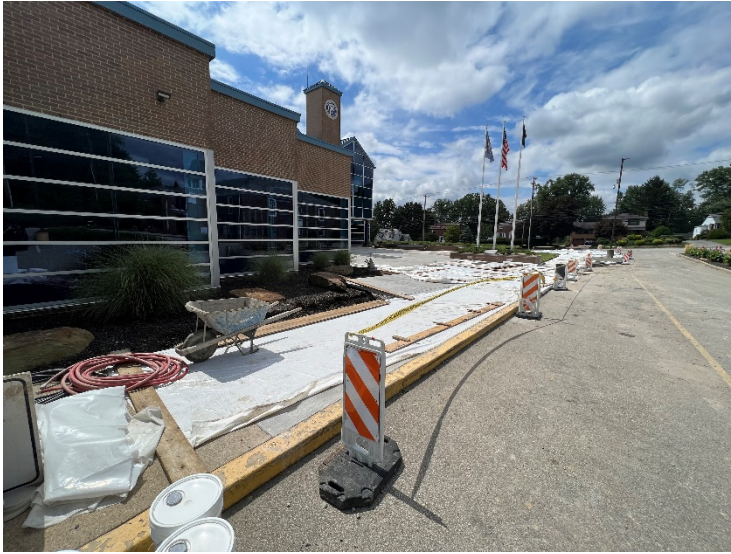
Existing entrance walkways have been replaced with new sidewalks.
